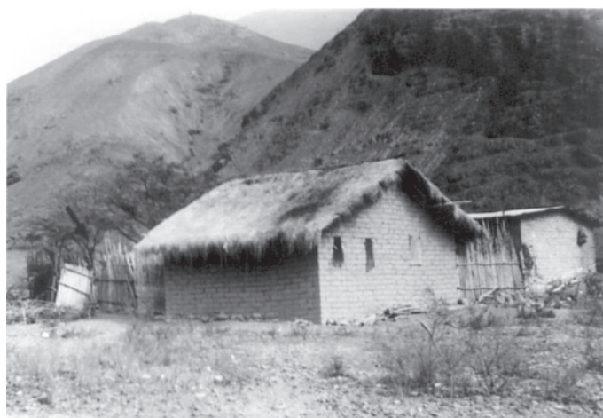
Fig. 2 - Typical example of household infested with Rhodnius ecuadoriensis : note the roof built with rice straw and non-plastered clay-bricks ("adobes") walls. At the peridomicile, an Cavia porcellus corral built with cane and clay ("quincha")- an ecotope for the specie.
