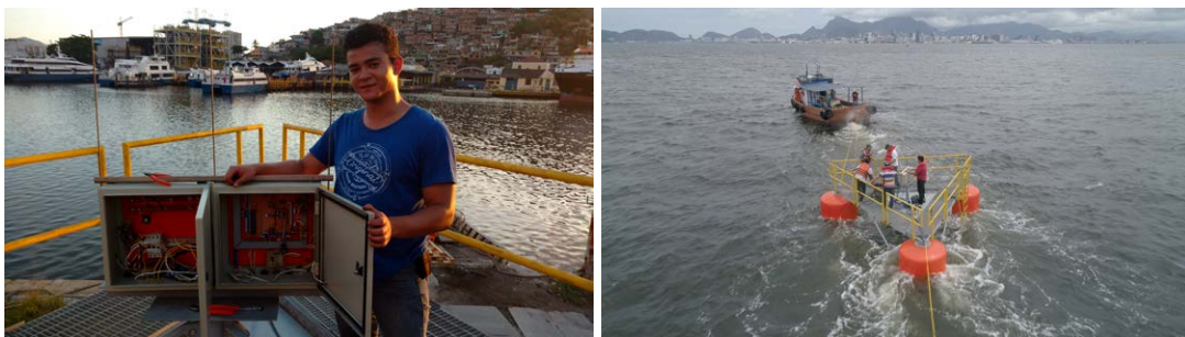
(a) Instrumentation platform installed on HK 3 -10 array (b) Test run of a HK-10 turbine with the instrumentation platform
