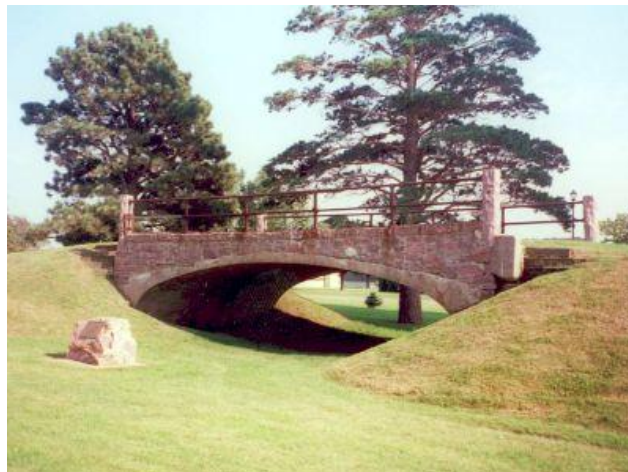
Figura 2.1- Rock Rapids Bridge (SMITH, 2013).
