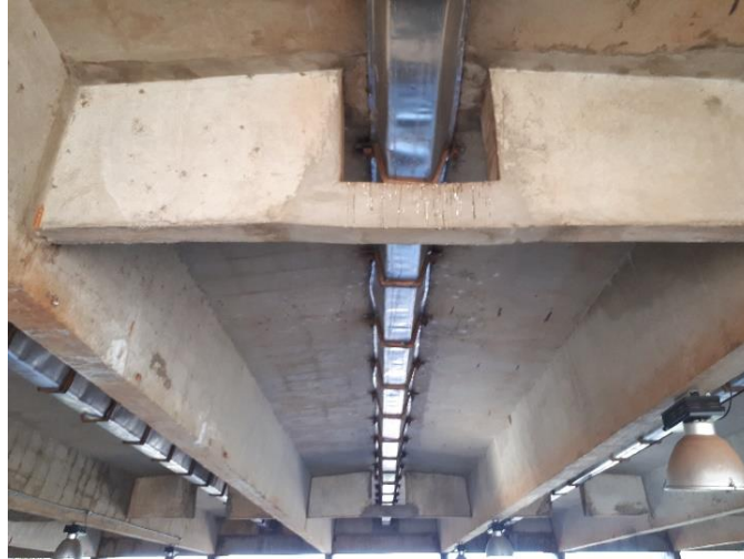
Figure 40: strengthening girders (private collection)
