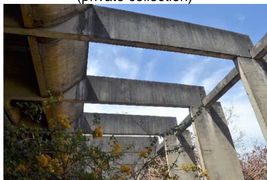
Figure 60: T-beam ends toward the internal pillars – section 588 - 594 (private collection)
