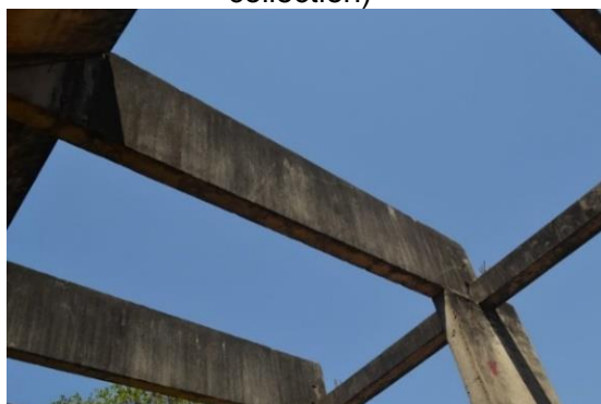
Figure 59: T-beam ends toward the internal pillars – section 516 (private collection)
