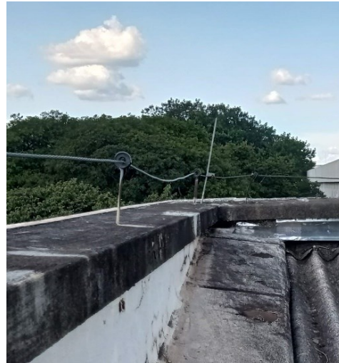
Figura 46 – Subsistema captor.
