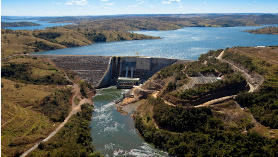
Figure 1.1 – Sefac hydroelectric facility, showing the dam with the upstream and downstream channels, with the downstream channel showing signs of a slight curve, suggesting heightened secondary flow in that area.
