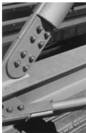
Figure 3.2 A bolted connection [94].
