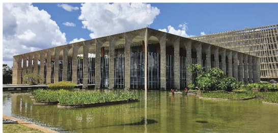
Figure 1. The external view of the “Palácio do Itamaraty”.
