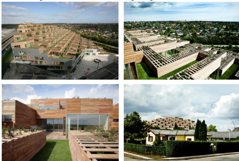
Figura 20 – Mountain Dwellings, Big Architects.
