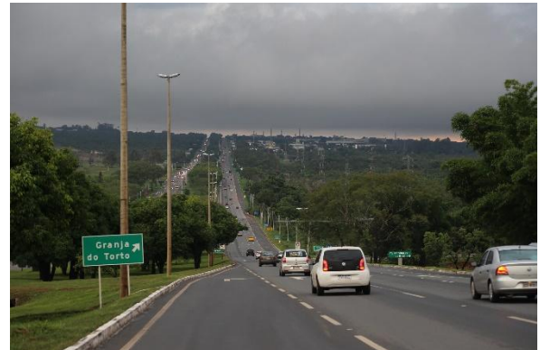
End of the section by the EPIA roadway that borders the CUB.
