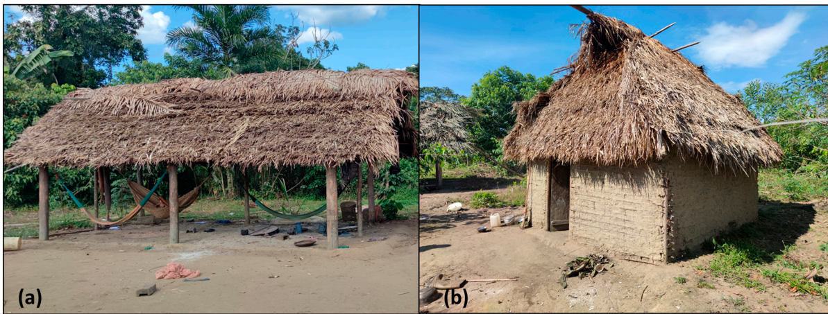
Figure 3. (a) House with no walls at all; (b) house with walls made from clay and sticks.
