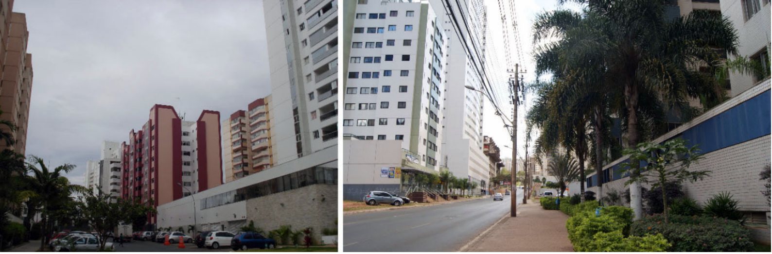
Figure 8: Photographs of a mix of streets and avenues in Águas Claras showing a profusion of occurrences of windowless façades. Source: author's personal file.
