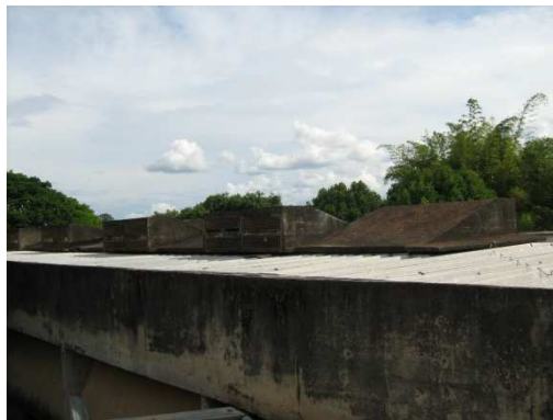
Figura 4.70 – Sheds de concreto
